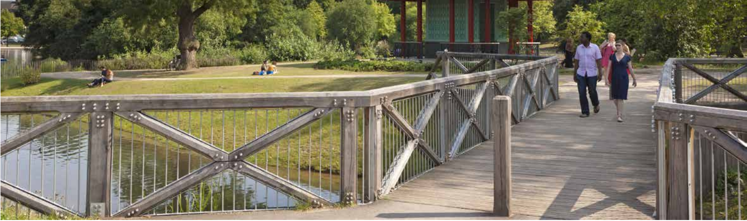
Victoria Park Footbridge (LDA Design)
